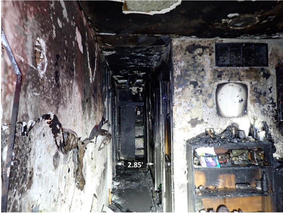
Figure 53. Hallway (looking towards Side Delta from the Living Room)
