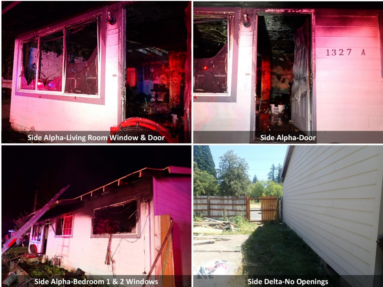
Figure 44. Ventilation Openings on Sides Alpha and Delta
