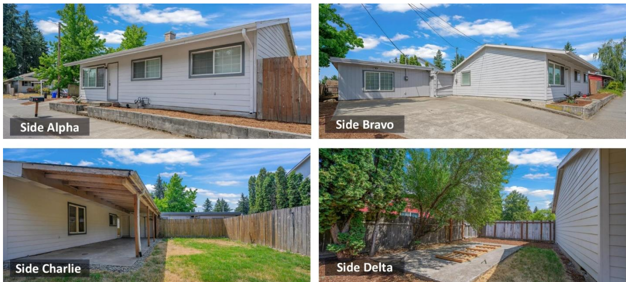
Figure 21. Building Exterior 1327 SE 182nd Ave #A.
