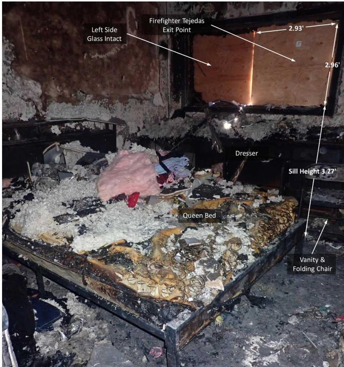
Figure 38. Bedroom 2 Exit Point
