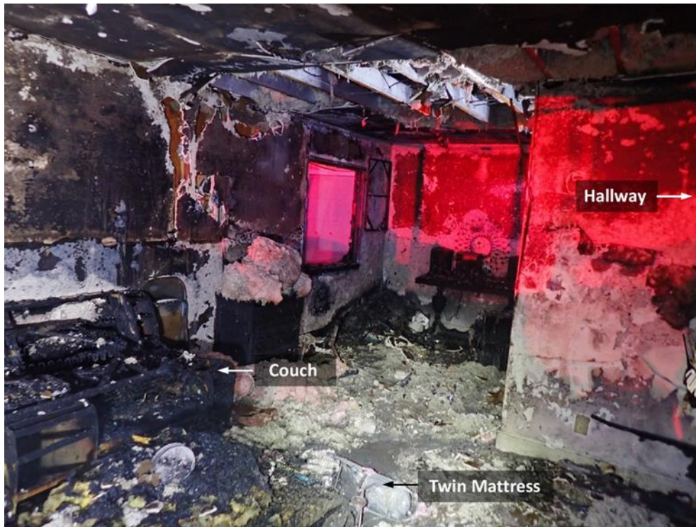
Figure 49. Living Room (looking towards the Bravo/Charlie Corner)
