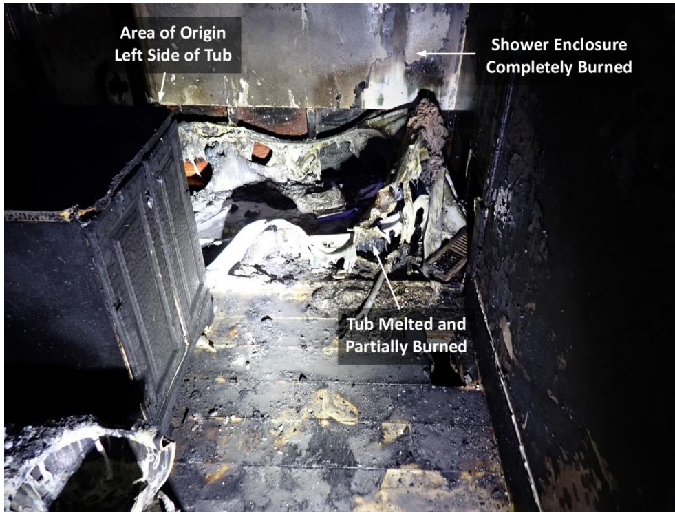
Figure 55. Bathroom (looking towards Side Charlie from the Hallway).
