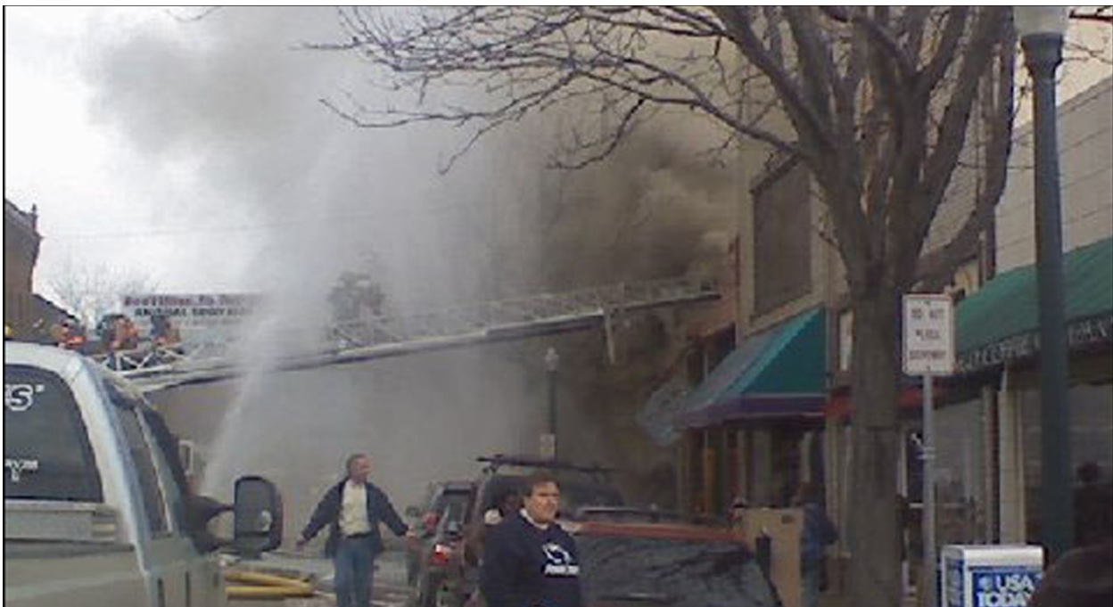
Figure 12. Conditions on Side A Immediately Following the Explosion.
