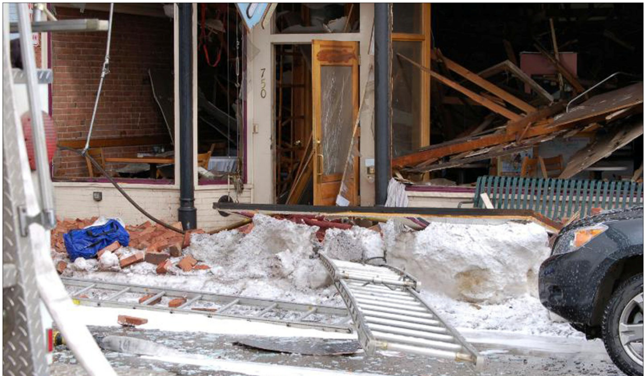
Figure 13. Side A in Front of Exposure D2
