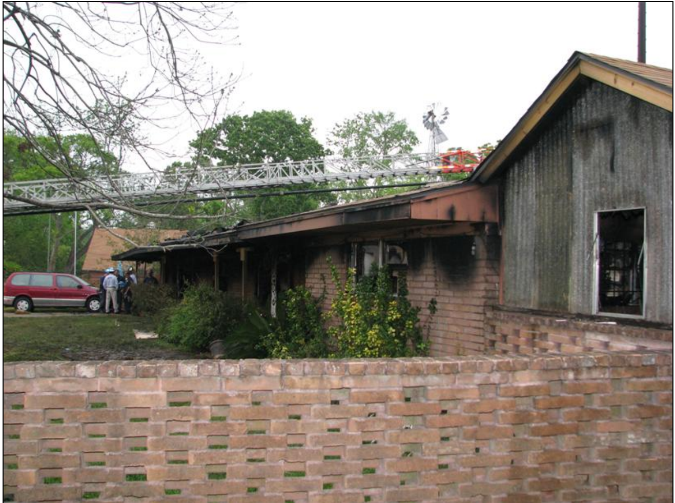
Photo 2: Photo taken from the A-D corner of the fire structure shows how access to the D-side of the structure was limited by the masonry wall. Photo provided courtesy of the fire department.
