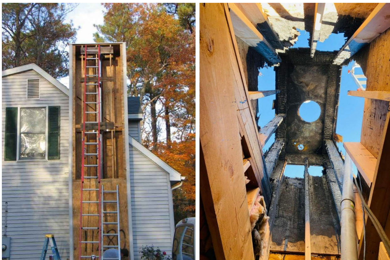
Figure 8. Wood Framed Chimney Chases
