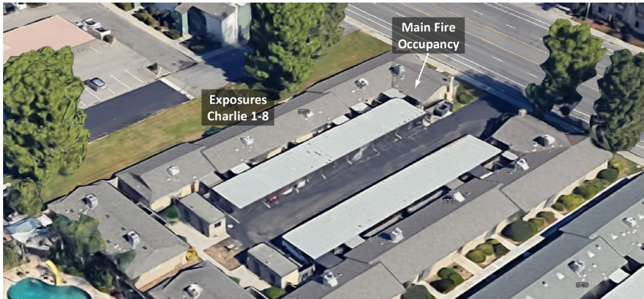
Figure 6. 3D Aerial View Bravo/Charlie Corner
