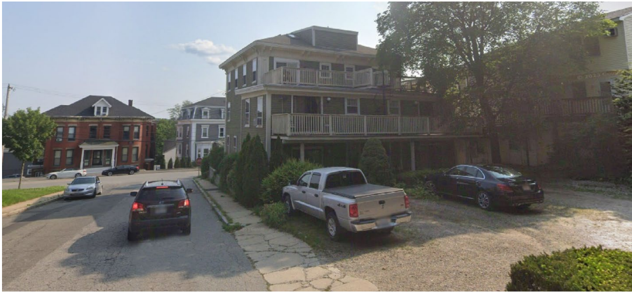
Figure 4. Charlie/Delta Corner from Webster Street
