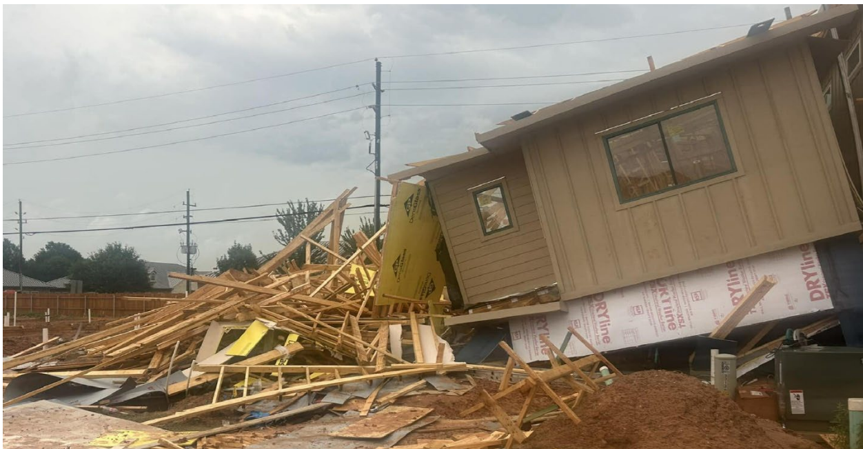
Figure 5. Conditions on Side Alpha
