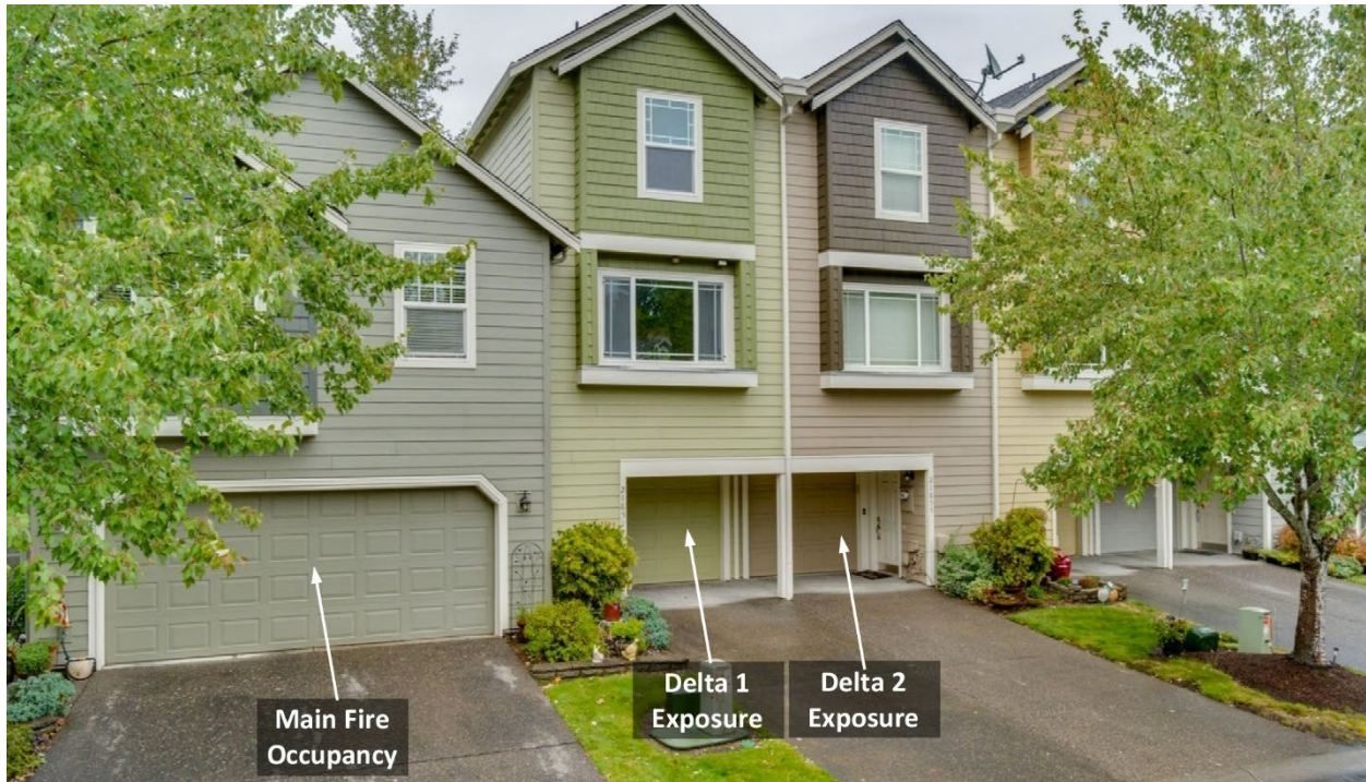
Figure 5. Side Alpha-Main Fire Occupancy and Delta Exposures
