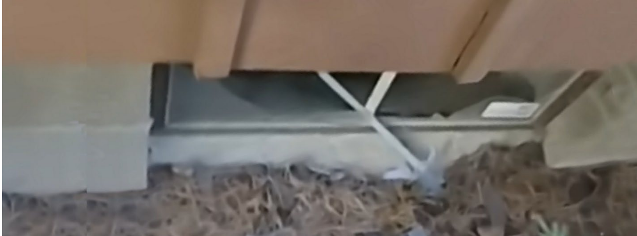
Figure 12. Lookout Basement Window
