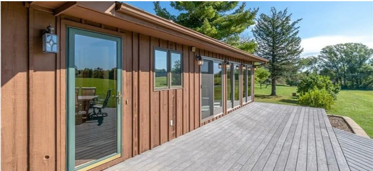
Figure 7. Side Charlie (Looking Towards Side Bravo)
