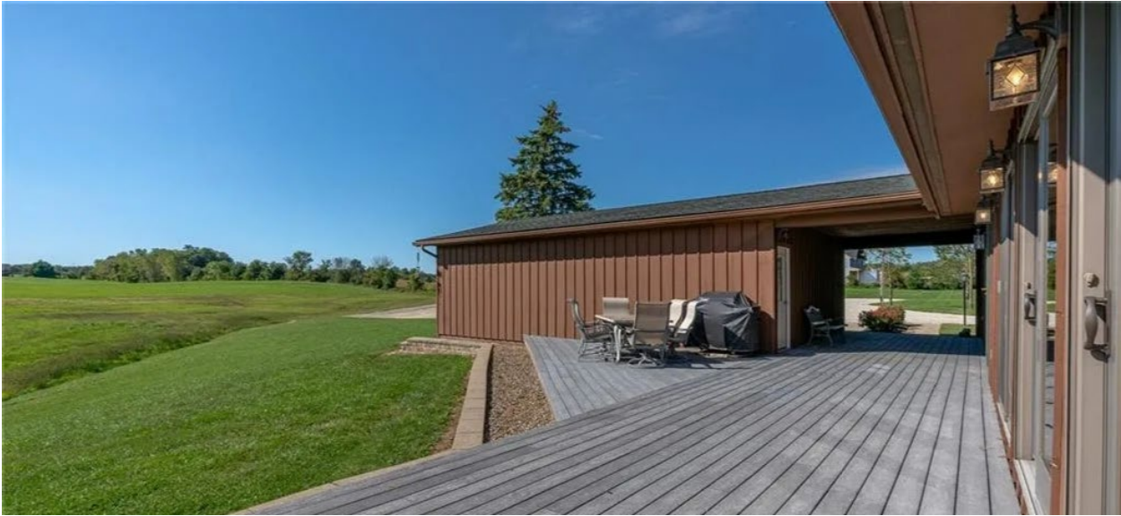
Figure 6. Side Charlie (Looking Towards Side Delta)
