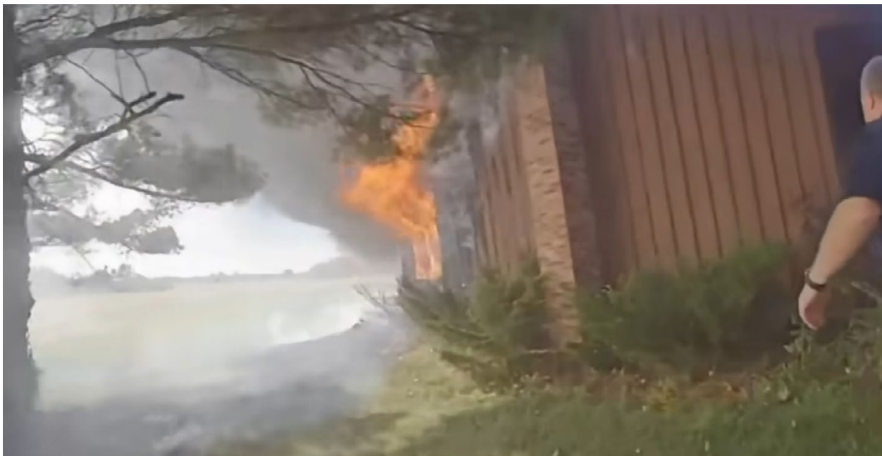
Figure 11. Condition on Side Bravo
