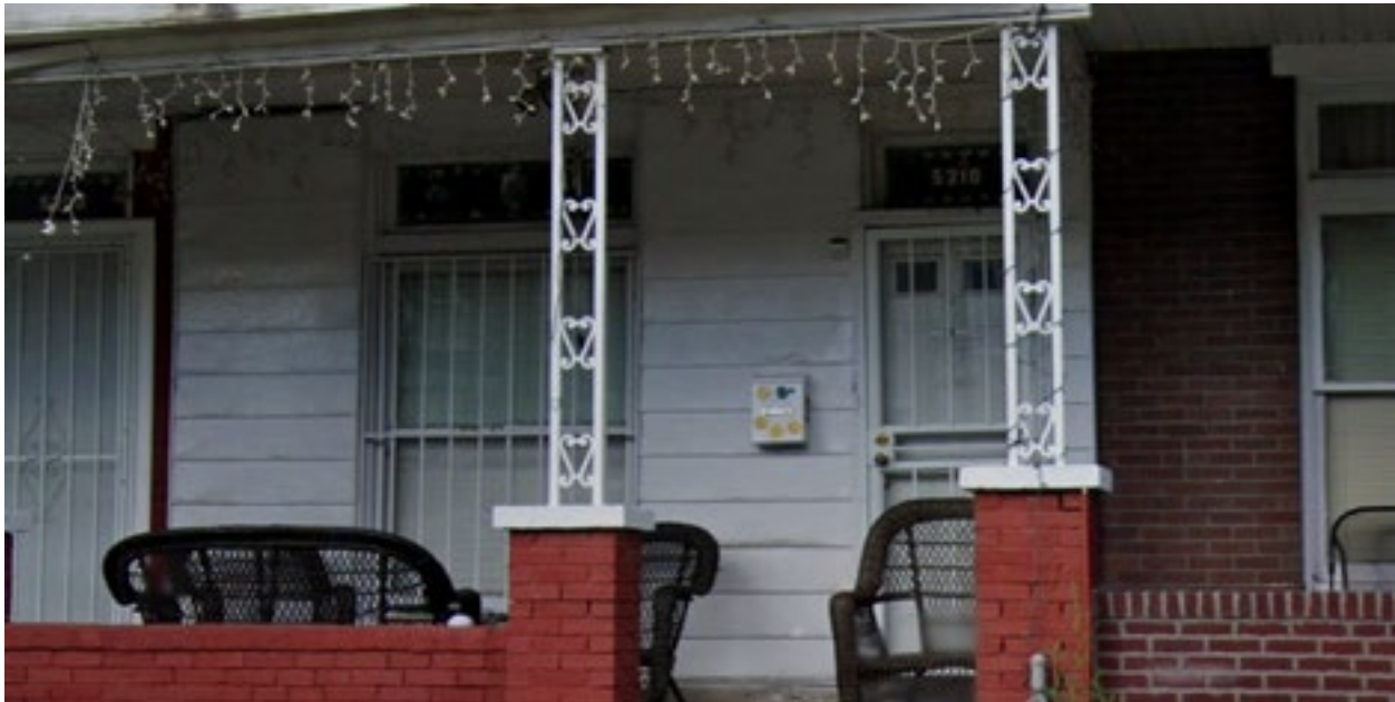
Figure 6. Security Bars on Side Alpha of the Main Fire Occupancy
