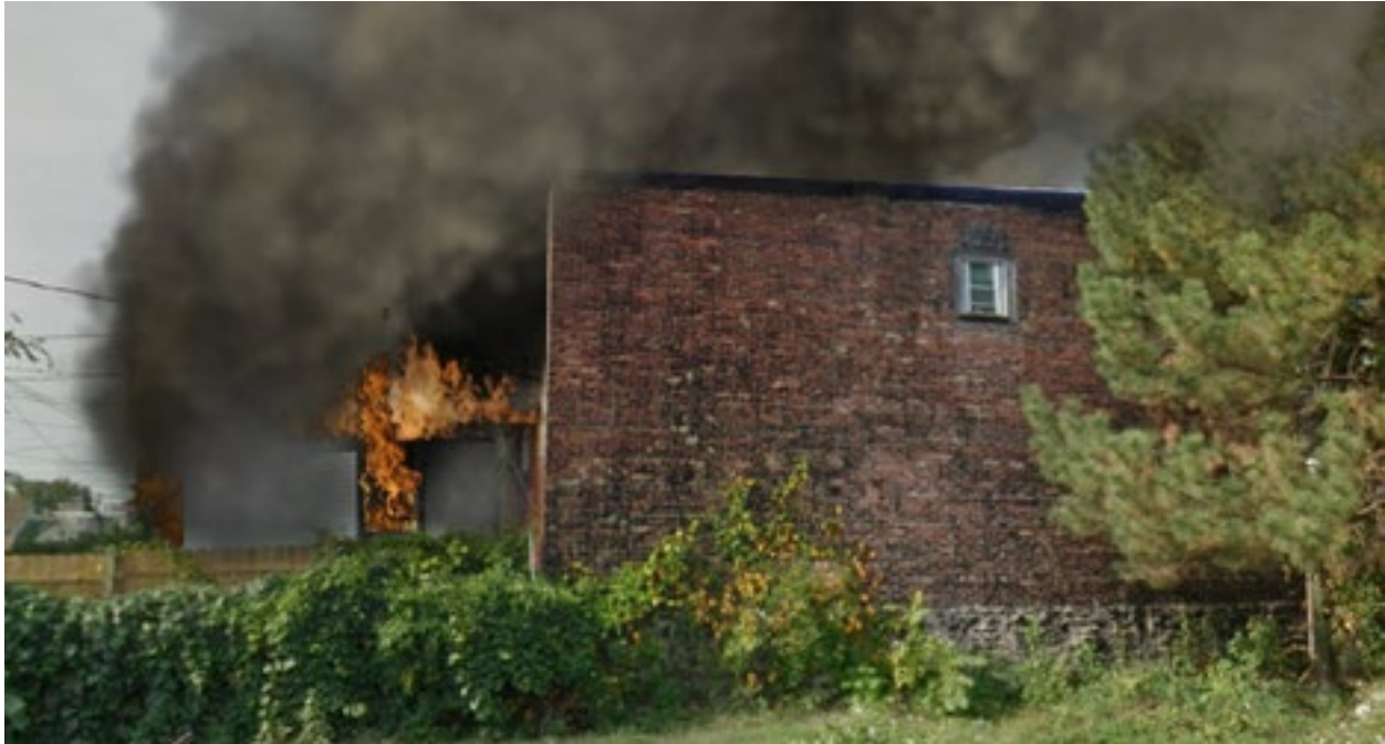
Figure 12. Conditions Visible from Side Bravo
