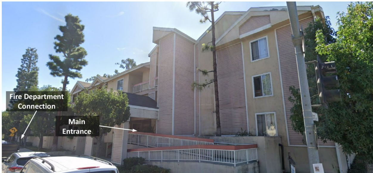
Figure 6. Side Bravo-Main Entrance
