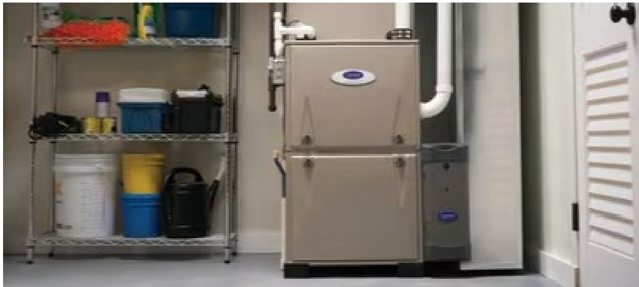
Figure 8. Forced Hot Air Furnace (representative example)
