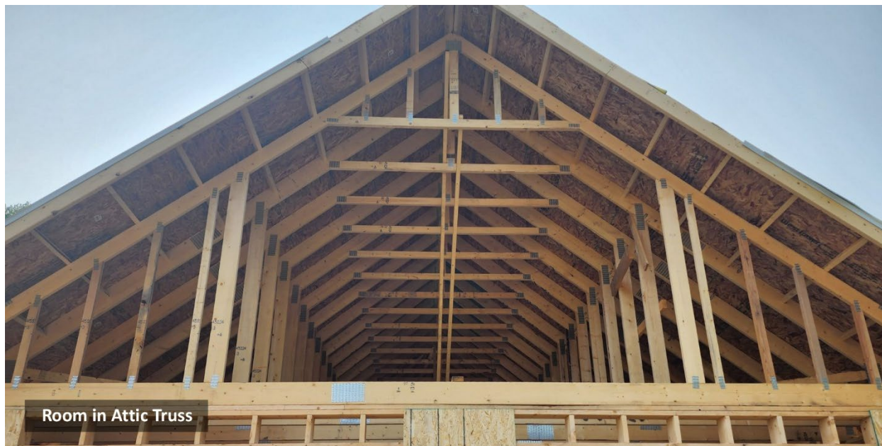
Figure 13. Room in Attic Truss
