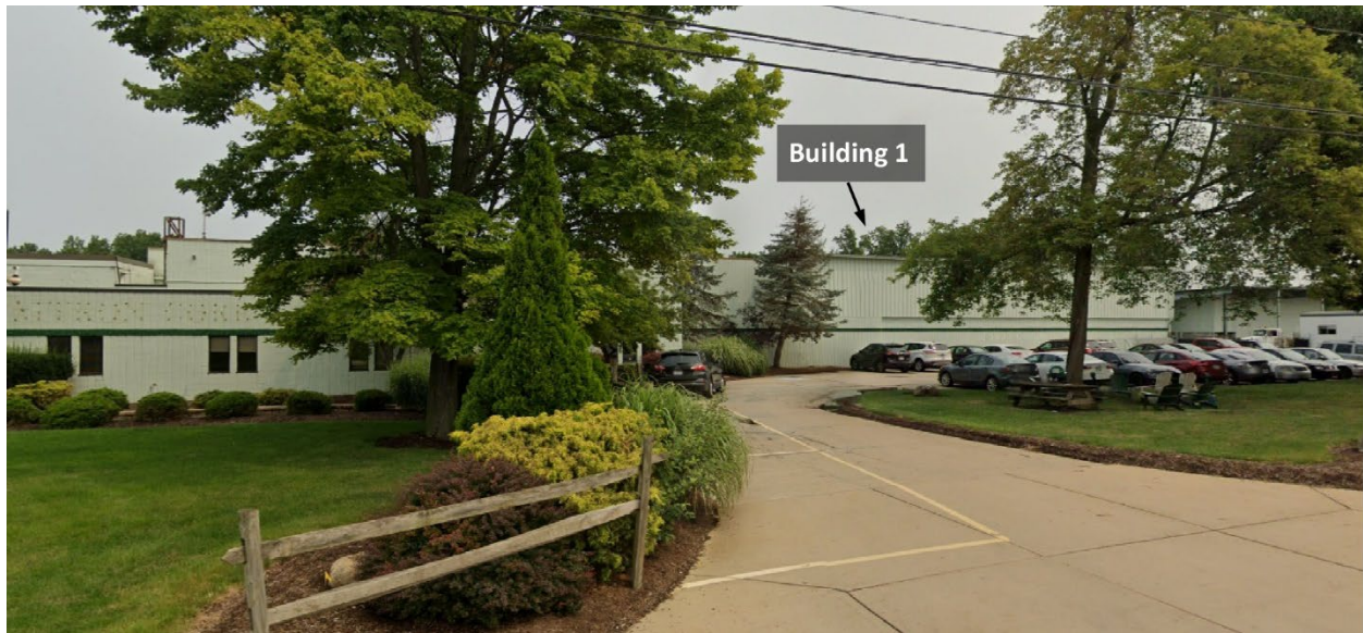
Figure 4. Building 1 Side Alpha
