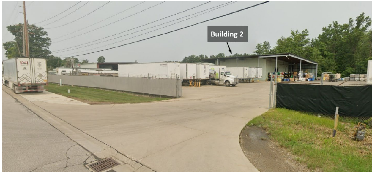
Figure 6. Building 2 Alpha/Delta Corner
