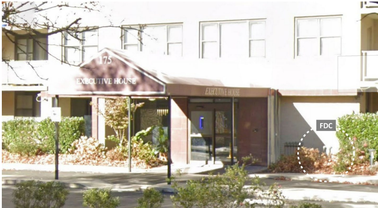
Figure 6. Side Alpha-Main Entrance
