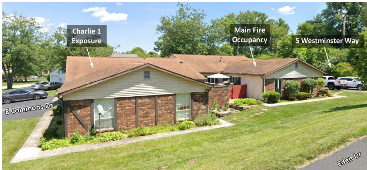
Figure 6. Side Bravo-Main Fire Occupancy and Charlie 1 Exposure
