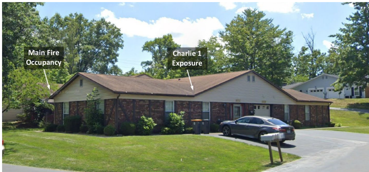
Figure 7. Charlie/Delta Corner-Main Fire Occupancy
