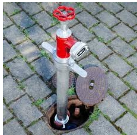
Figure 3. Underground Hydrant
