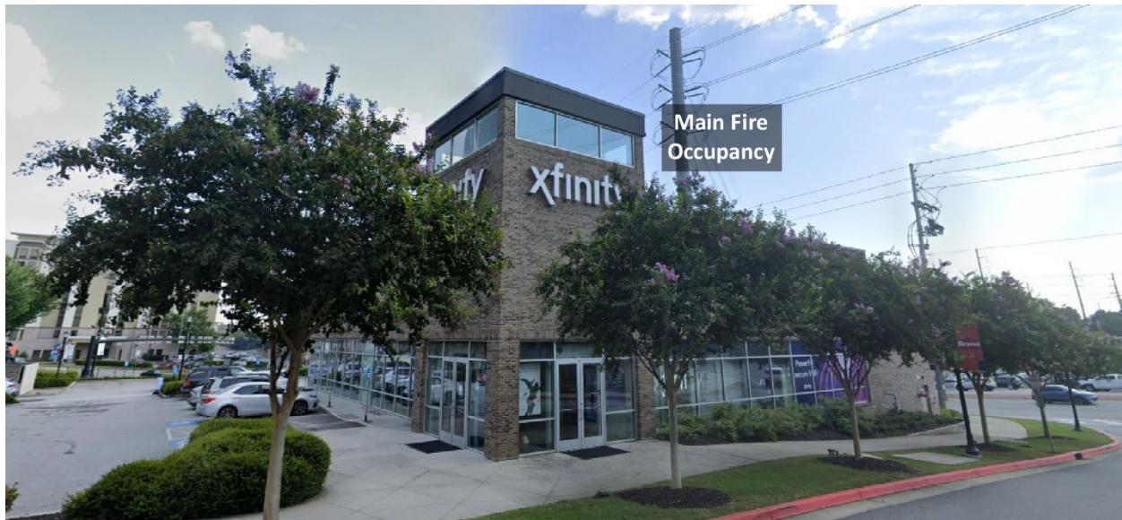
Figure 4. Alpha/Delta Corner (View from Relay Drive)
