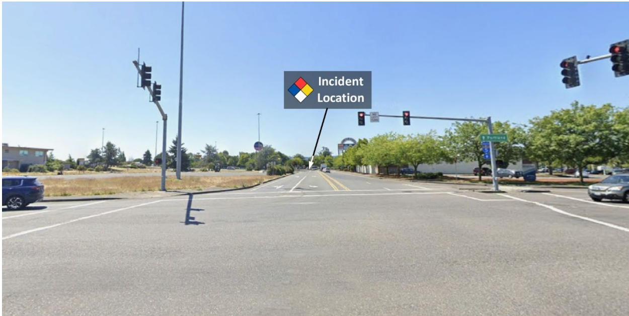
Figure 4. Northbound on North Center Avenue
