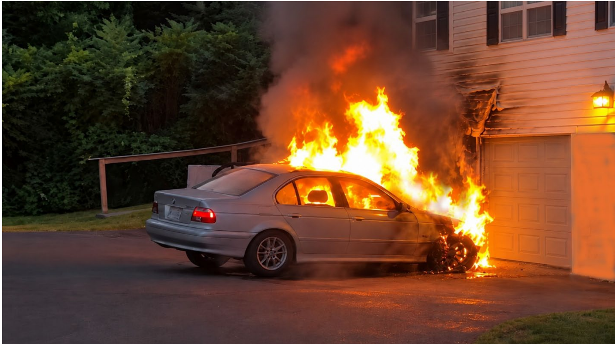
Figure 7. Close View of the Vehicle Fire and Thermal Damage to the Building
