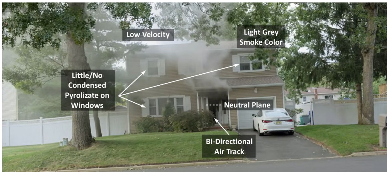
Figure 7. Reading the Fire at 75 Melody Avenue
